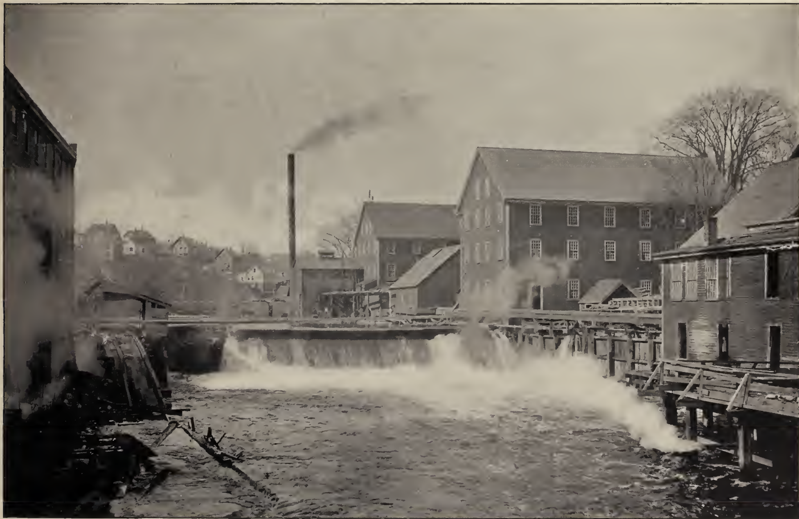
DAM NO. 2, OWNED BY JOSHUA GRAY—FALL. 12.50 FEET. See Page 99.
